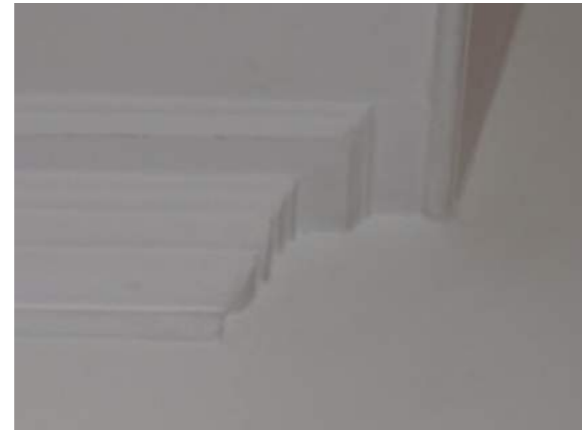
Moulded cornice detail abutting stair
