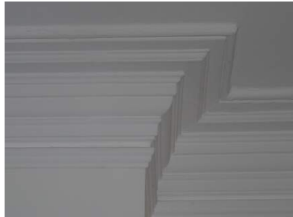
Moulded cornice detail to the ceilings
