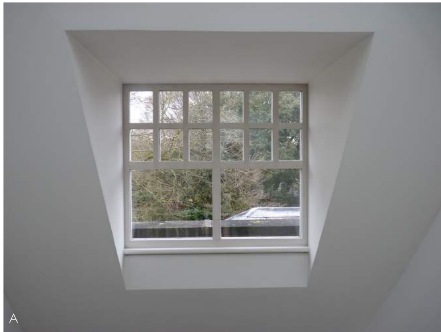
Photos A-D These photos show typical door architrave detail, simple skirting boards to all rooms and various modern dormer windows.
