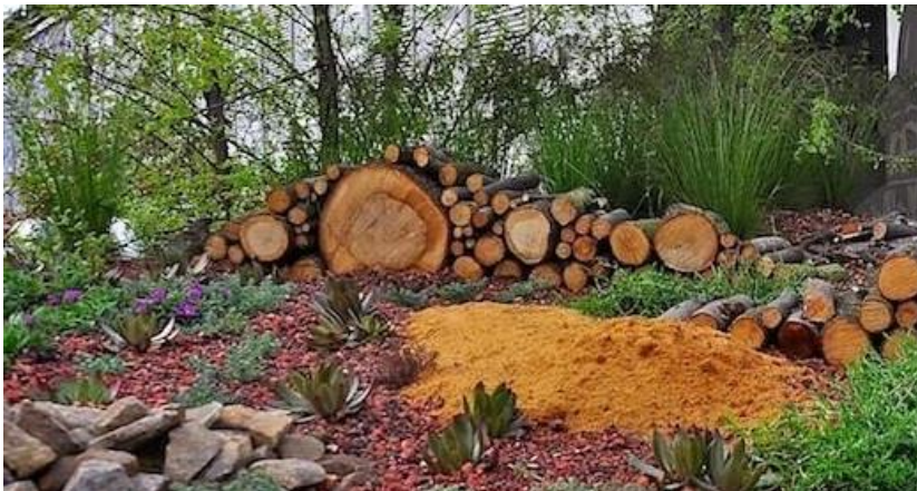
Figure 6.3 Log and sand piles on a biodiverse roof
