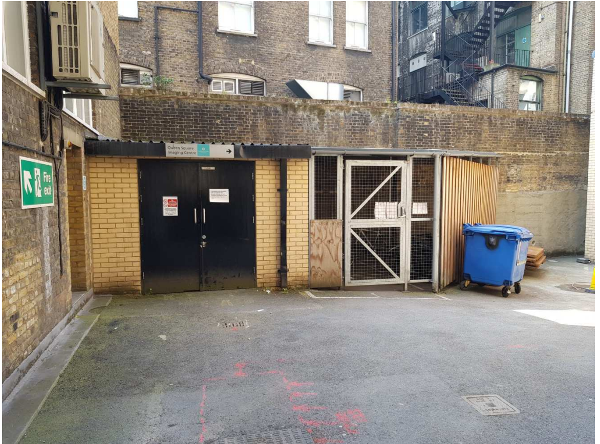
Figure 2. External view of the current medical storage and cycle store, chosen for the location of the substation.
