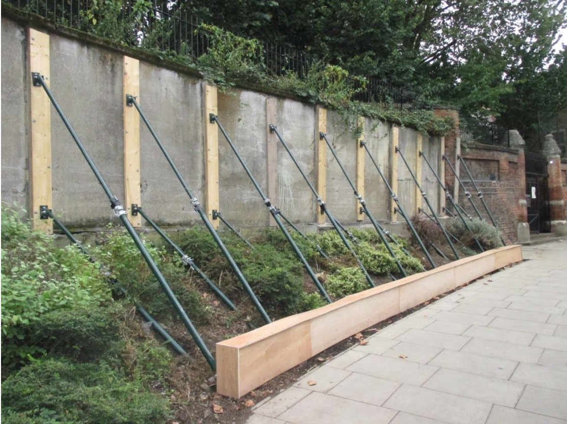
Photo 2 – Supports to the retaining concrete wall installed in August 2016
