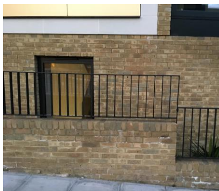
Figure 7 - Example flat infill bar railings
