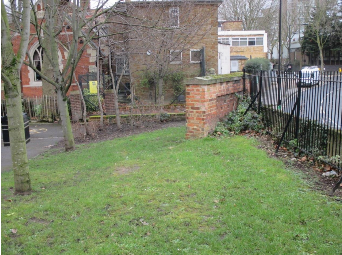
Photo 4 – Close view of the area of work
