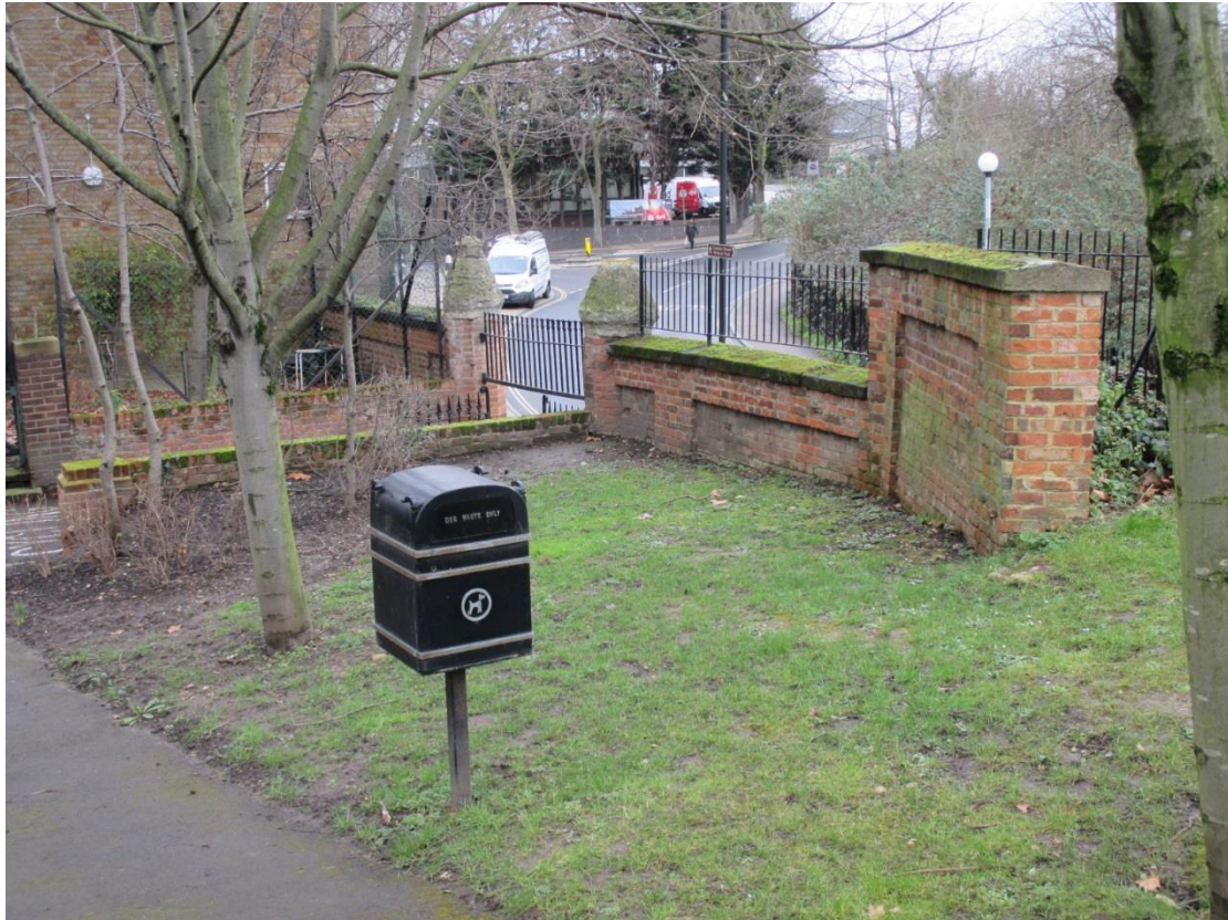
Photo 5 – Existing brick retaining wall
