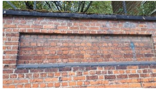
Figure 3 - Existing brick wall
