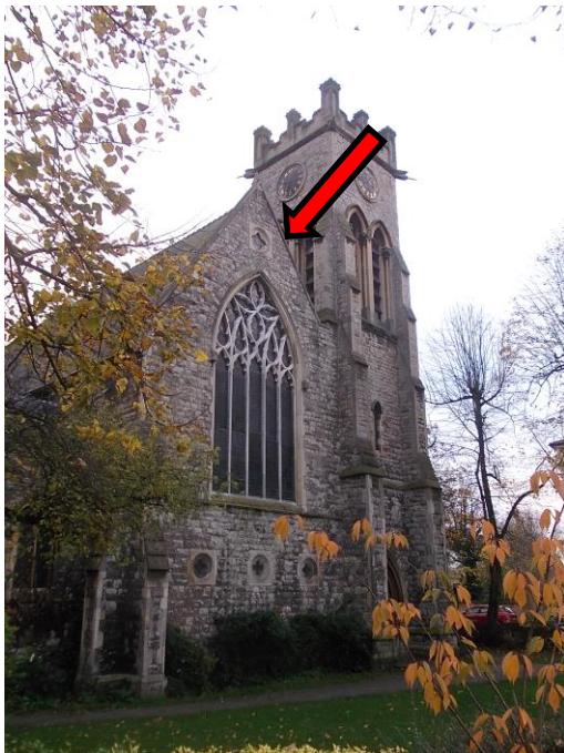
Location of Belfry opening to be altered to give access to valley gutter
