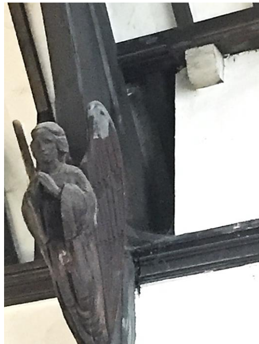
Timber angel corbel beneath valley gutter where leaks occur
