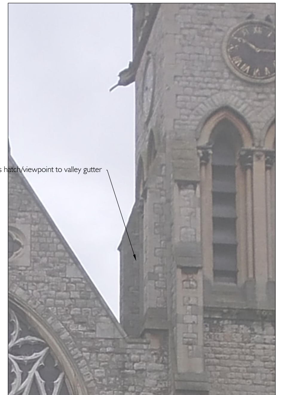
West elevation showing location of proposed access to valley gutter by inserting a hatch in place of the bottom louvre
