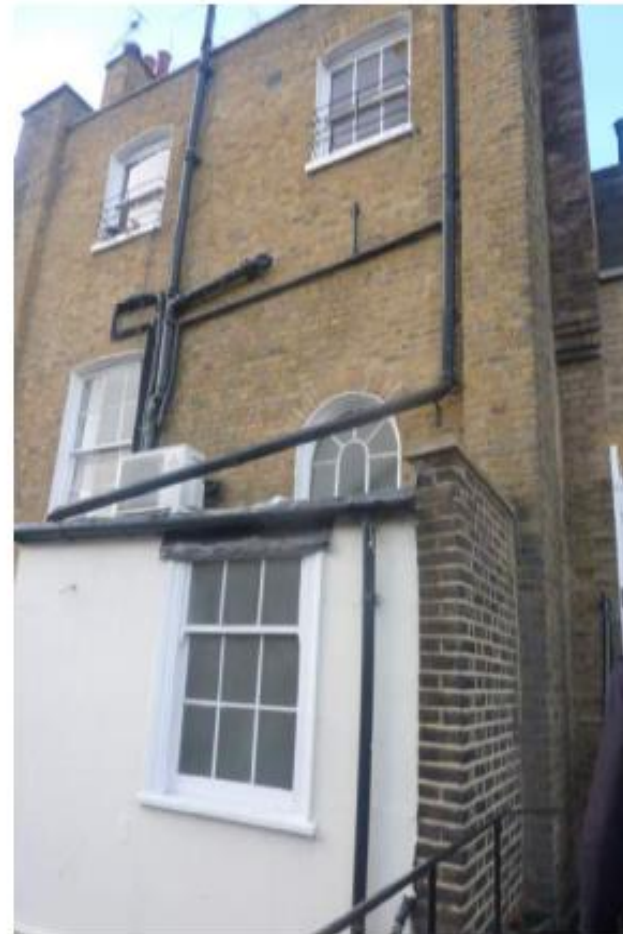
19 John Street Rear closet wing
