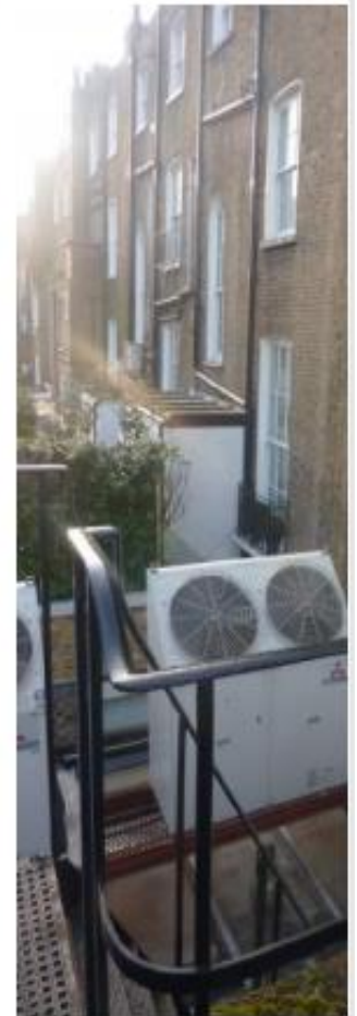
19 John Street Rear of property
