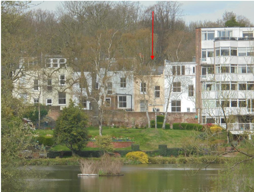
Photo 4 and 5 view towards the rear elevation form the opposite side of Hampstead Ponds
