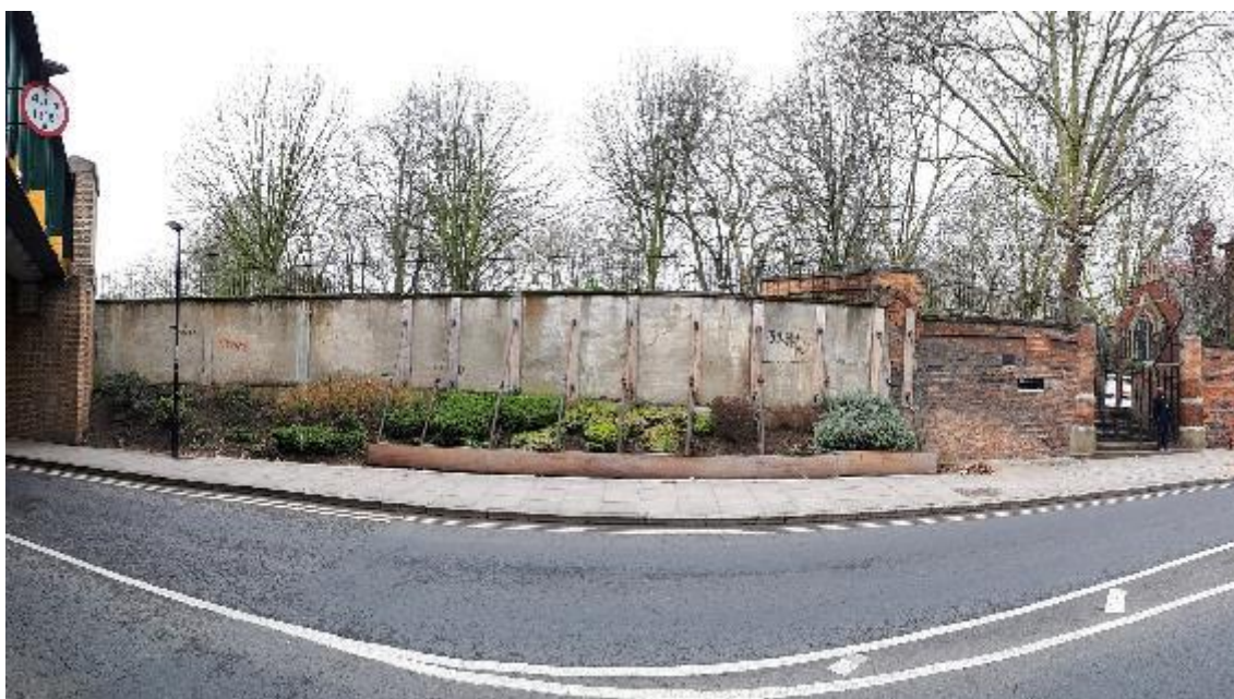
Photo 5 - Panoramic photo of the concrete wall currently supported since August 2016 (March 2019)
