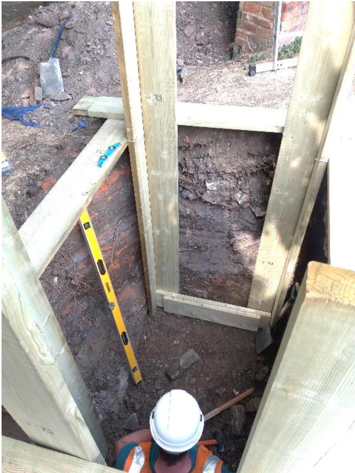
Photo 7 - 3m deep TP2 and original brick boundary wall (July 2017)
