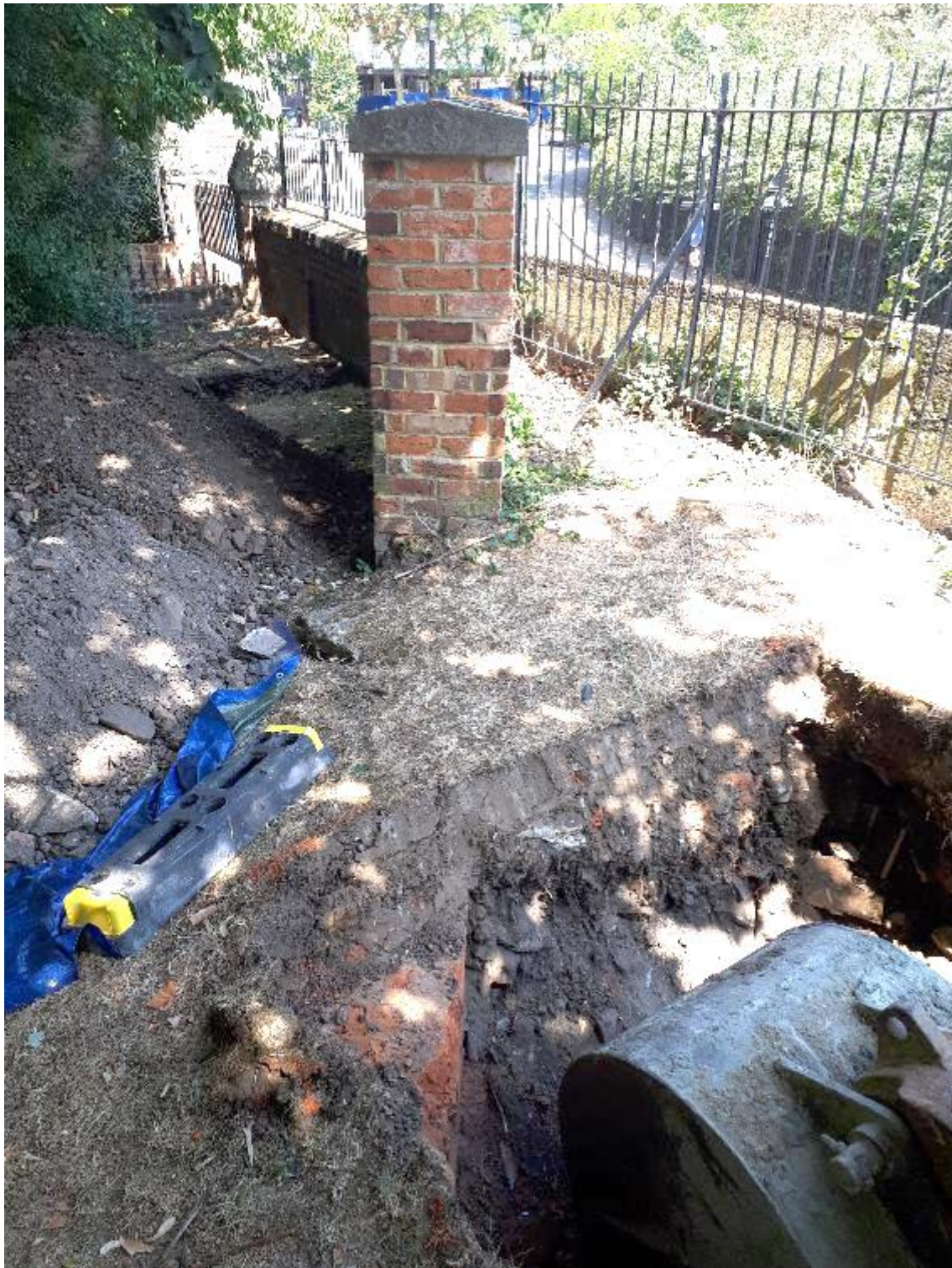
Photo 6 - Continuity of the original brick boundary wall below ground level at the TP2 (July 2017)
