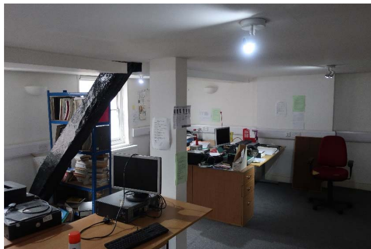
Third Floor office
