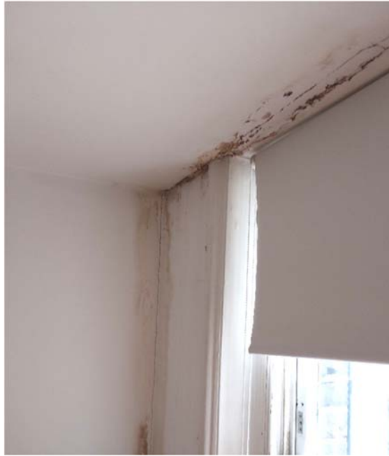
Leak to rear Second Floor wall
