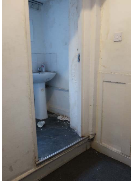
WC off stairwell at half level
