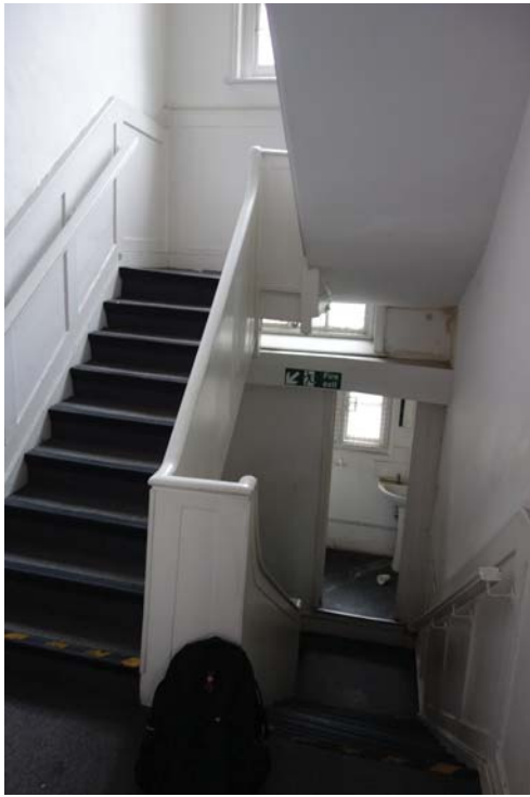
Photograph 12: view looking south-west of staircase
