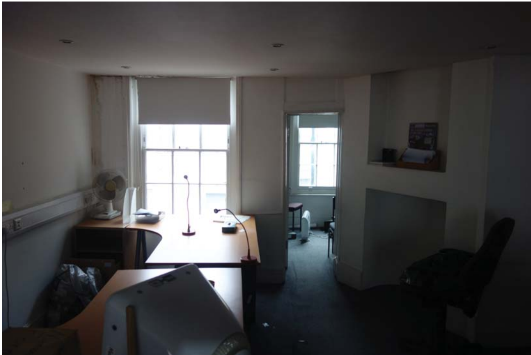
Photograph 16: view looking south-west across the rear office on the second floor
