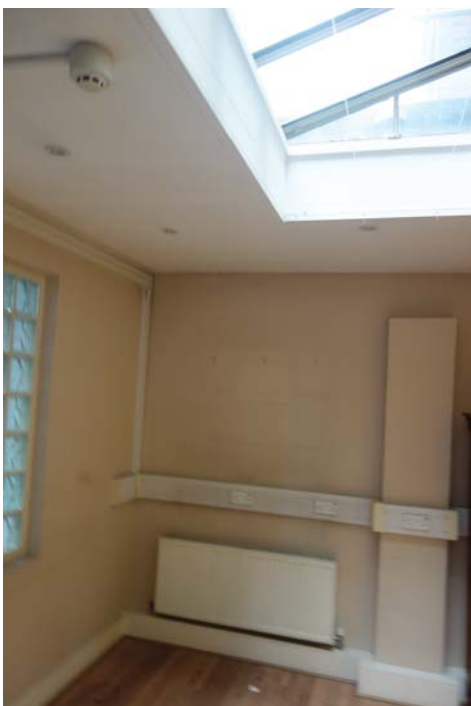
Photograph 8: view looking west of rear single-storey extension
