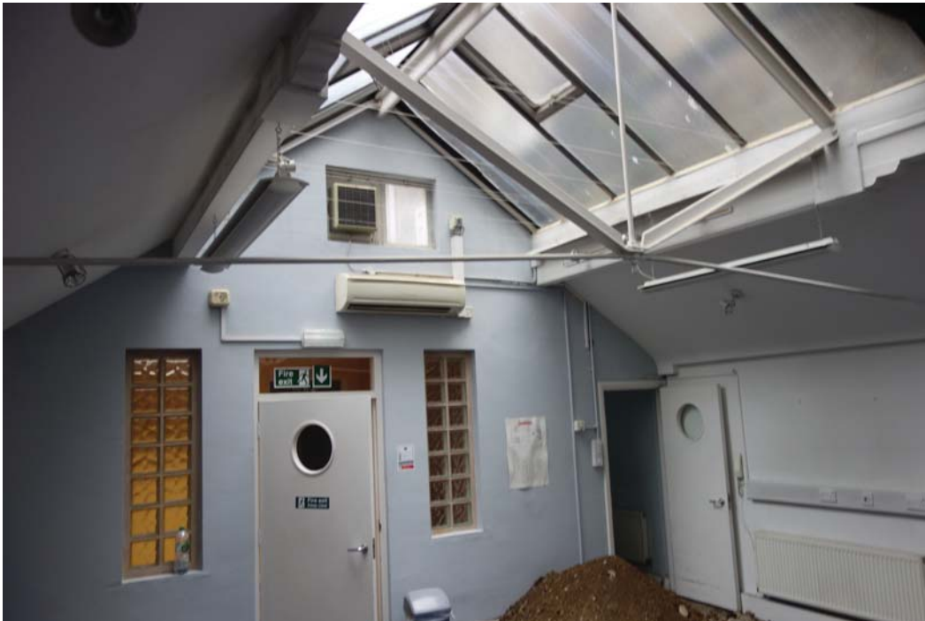
Photograph 7: view looking east of rear single-storey extension
