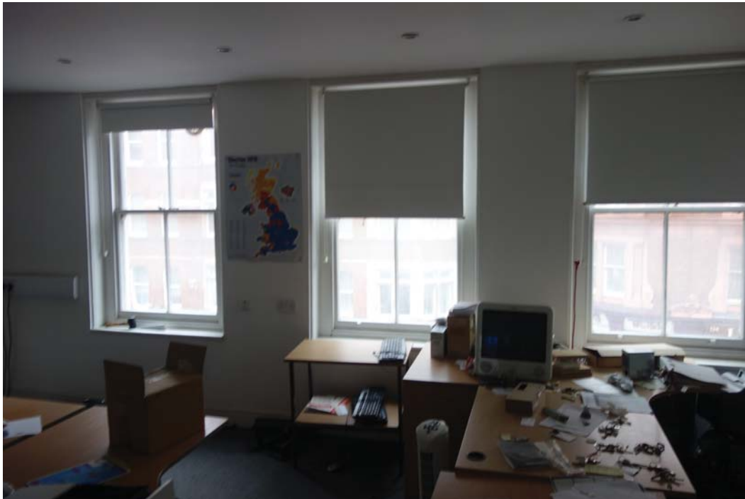
Photograph 14: view looking east towards the street frontage windows on the second floor front office
