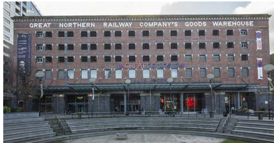
Solid facade, punched openings
