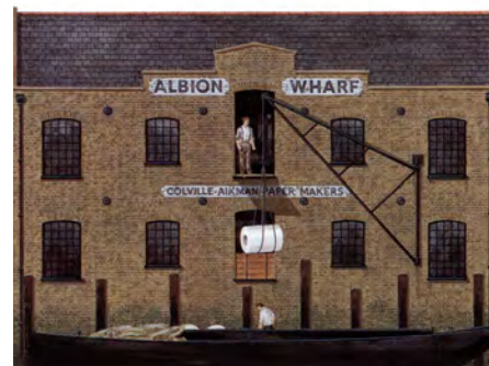
Solid facade, punched openings
