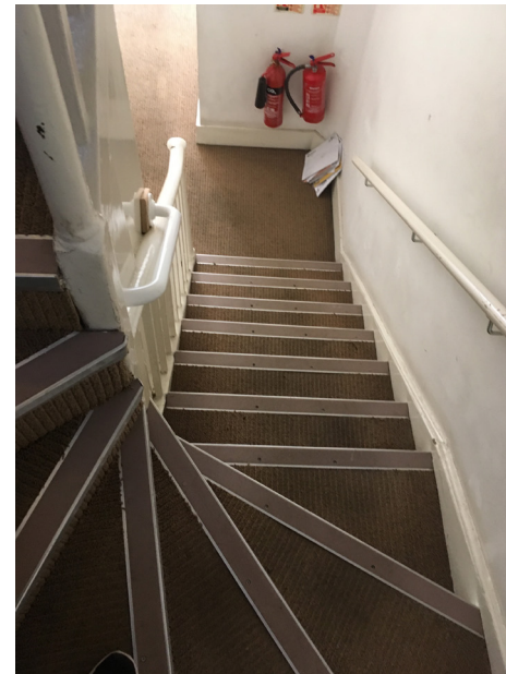
Original balustrading to stair to have paint stripped back and new painted finish.
