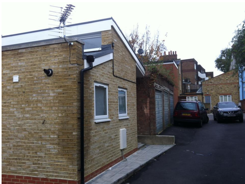
Residential Unit to rear of 104 Fortune Green Road, looking North
