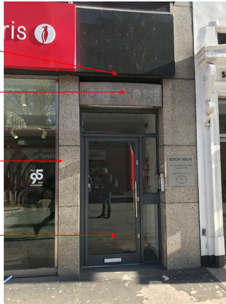
Existing Main Entrance to 177-178
