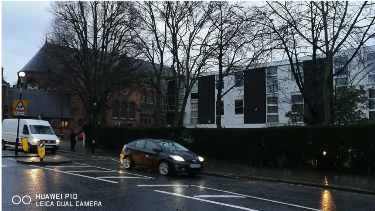
View from Primrose Hill_PV panels installation works stalled
