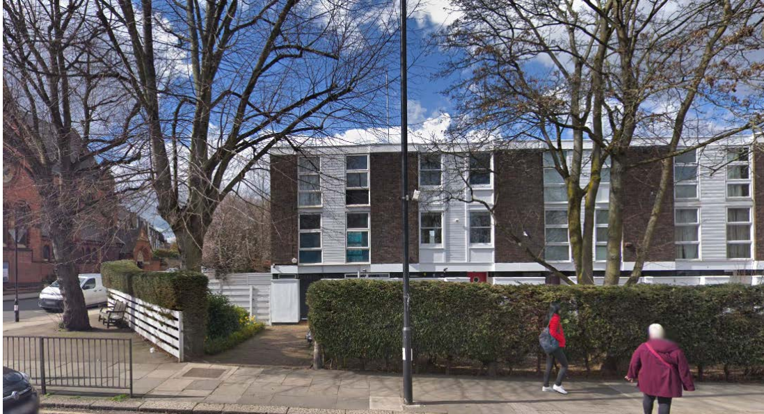
Front Elevation of No 11 Primrose Hill Road.
