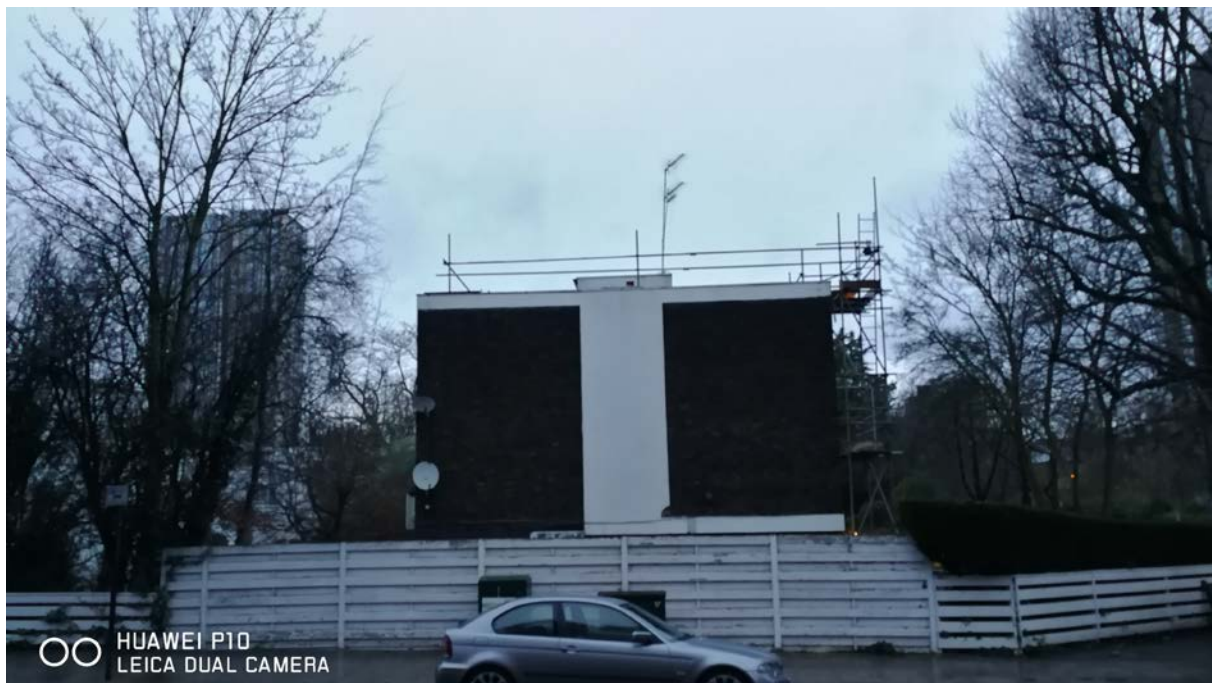
View from King Henry's Road_ PV panels installation works stalled
