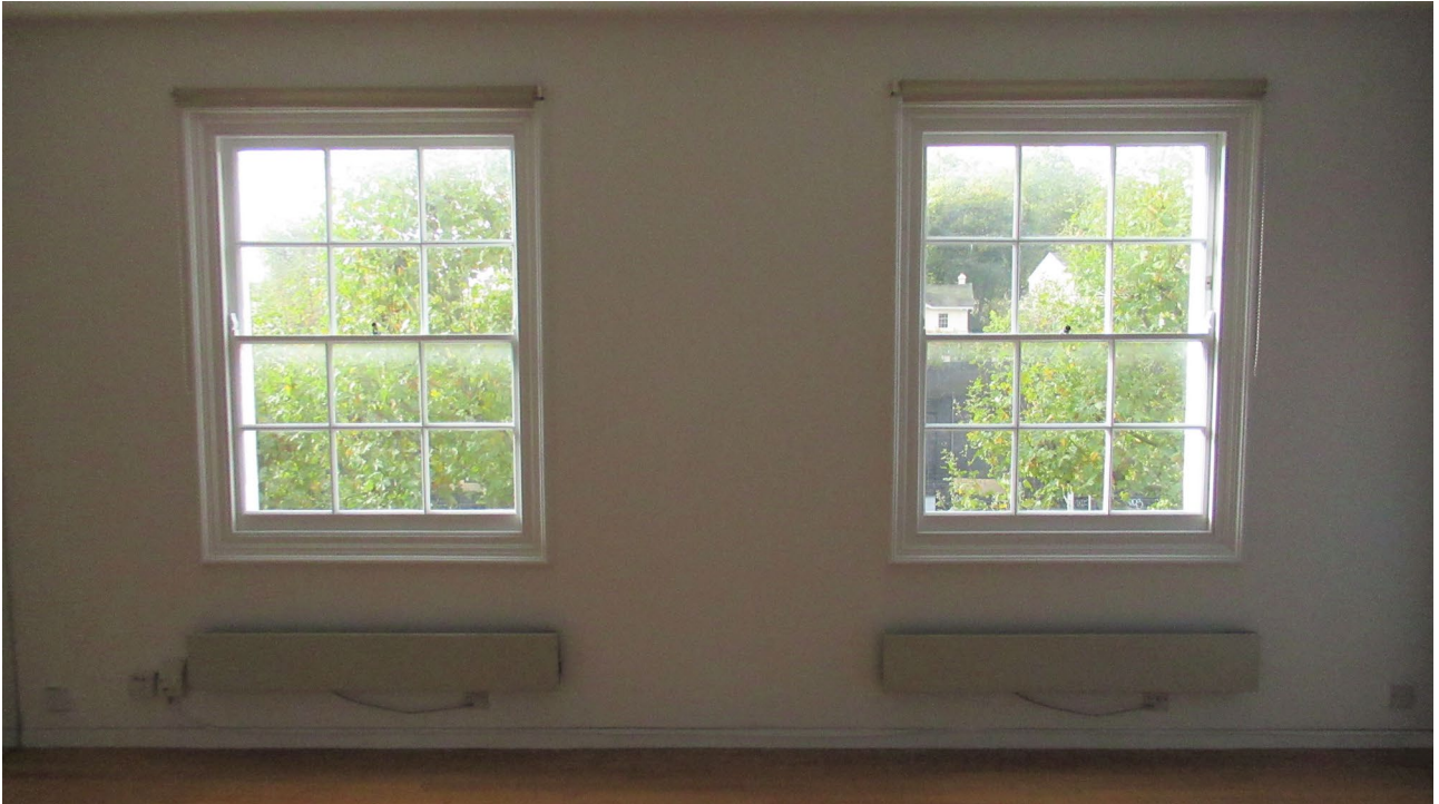
Figure 5: Internal view of two windows at second floor studio (Flat 4)
