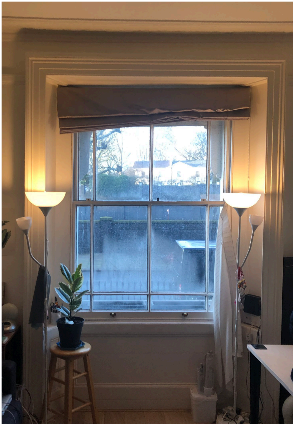
Figure 4: Internal view of window at ground floor lounge (Flat 2)
