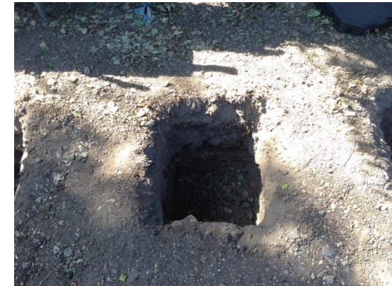
Fig 5 – Sample excavations for similar projects where careful hand digging is used and pad locations manipulated to reflect the presence of any root >25mm in diameter.
