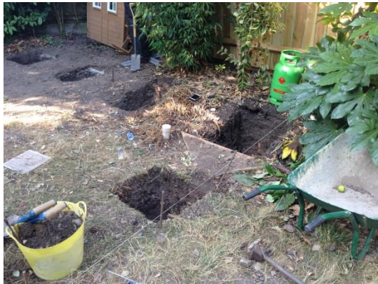
Fig 5 – Sample excavations for similar projects where careful hand digging is used and pad locations manipulated to reflect the presence of any root >25mm in diameter.
