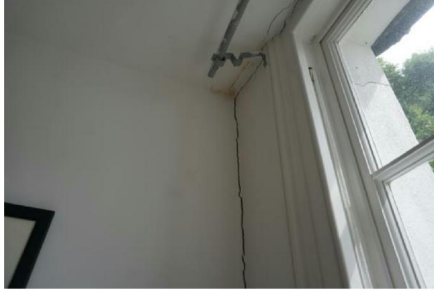
Stairs - Vertical crack at rear left junction.
