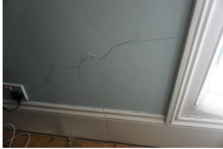
Front Bedroom - Diagonal crack.
