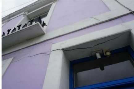
Front Elevation - Horizontal Crack.
