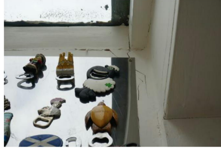
Dining Room - Tapering crack at main house junction.
