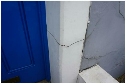
Front Elevation - Horizontal crack to right of door.
