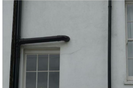
Rear Elevation - Horizontal Crack.
