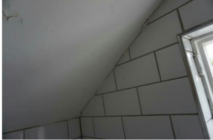
Bathroom - Ceiling junction separation.
