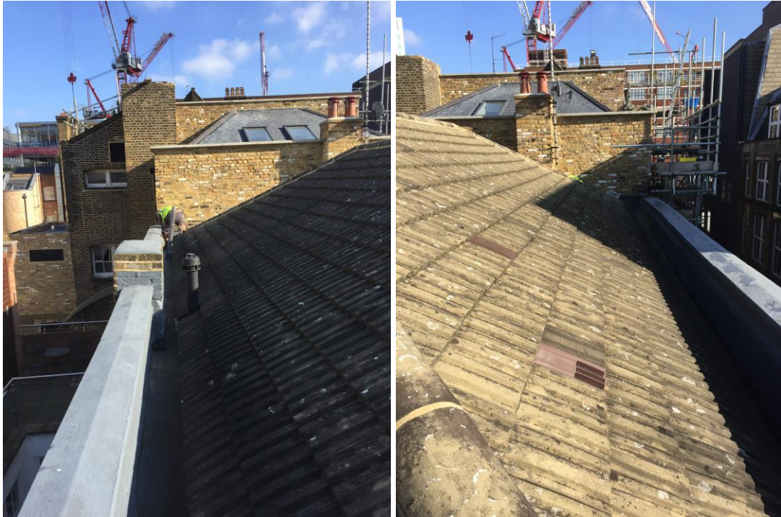
Existing raised party wall with nr 7 Midford Place
