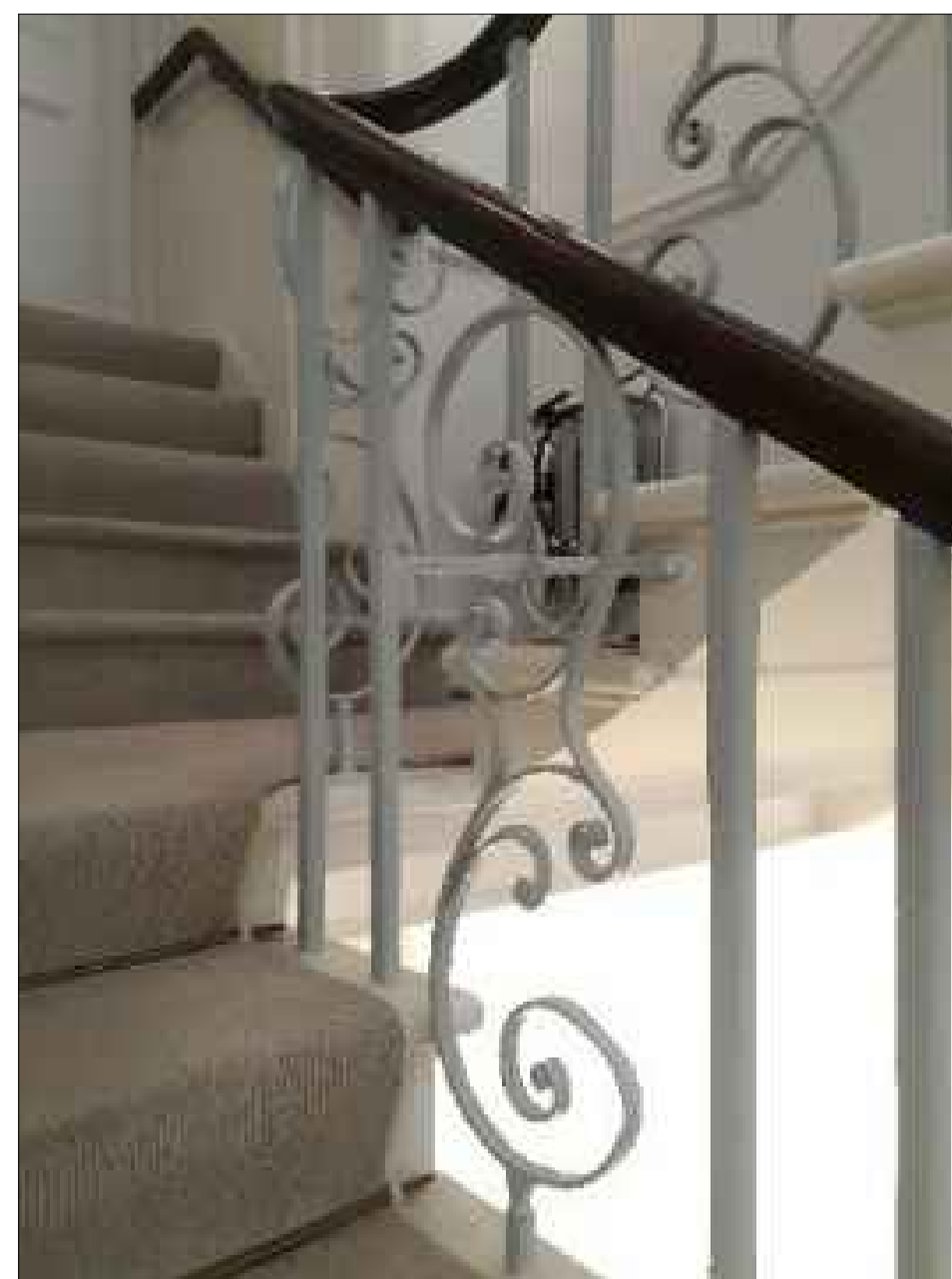
EXISTING HANDRAIL TO SC1
