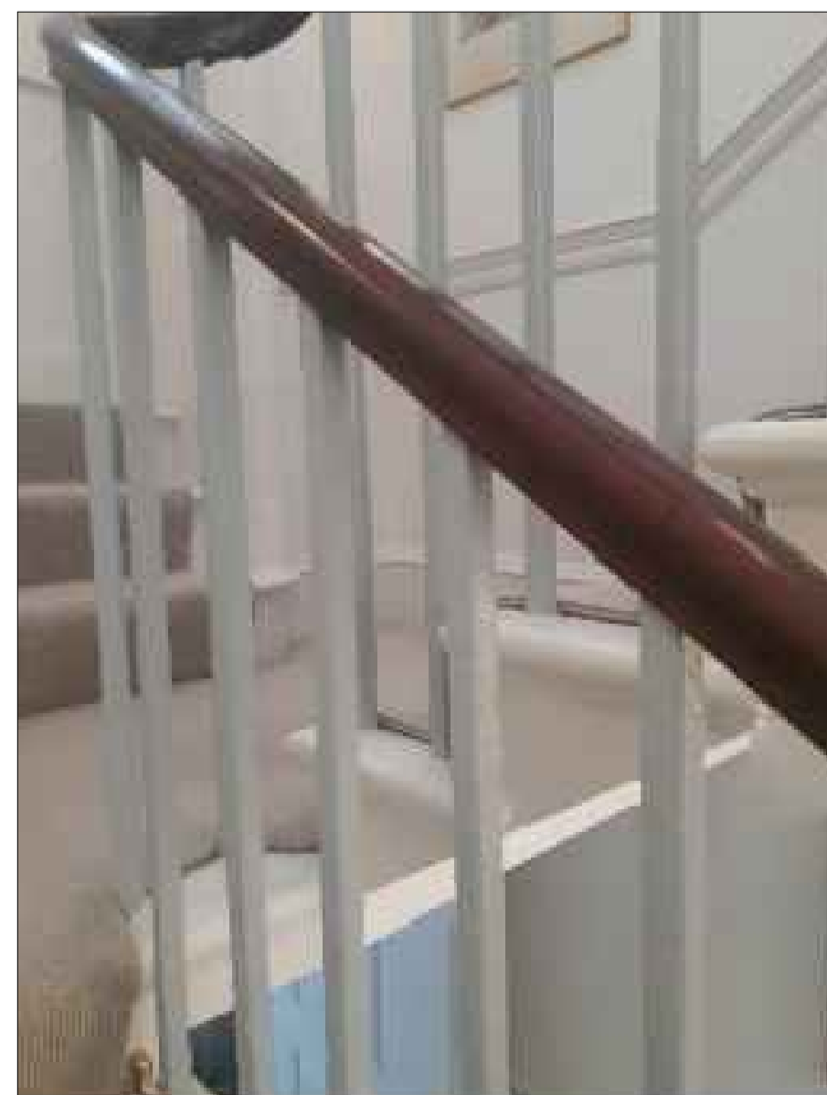
EXISTING HANDRAIL TO SC3
