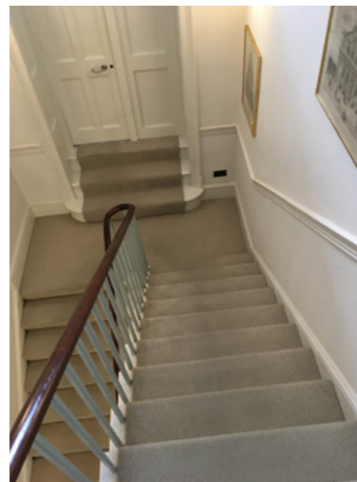
Existing stairwell of no.15: sc2 (first floor looking down)
