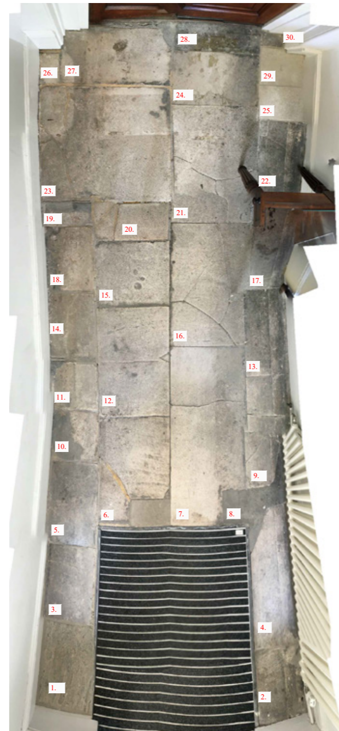
Photograph of existing floor
