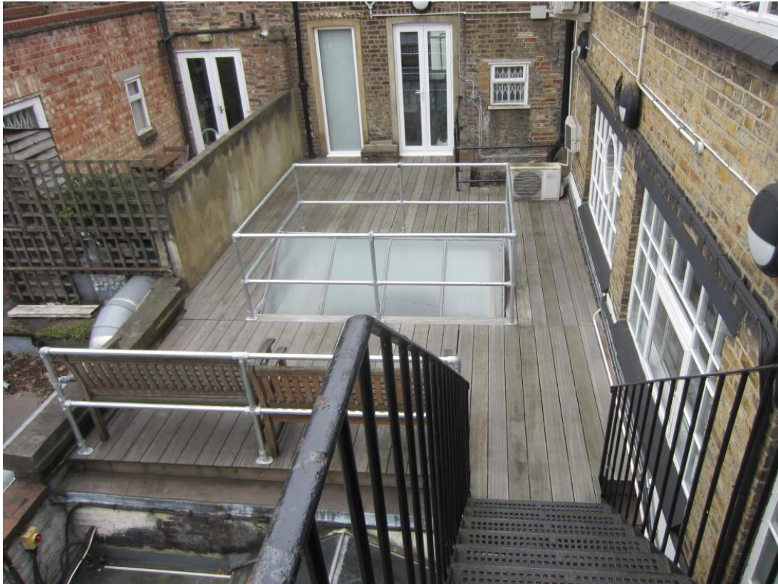
REAR VIEW OF FLAT ROOF OVER RESTAURANT – USED FOR EMERGENCY ACCESS BY OFFICES
