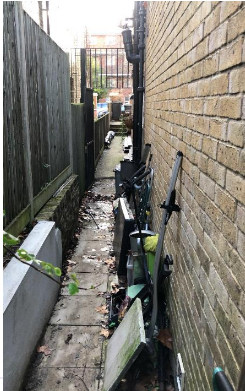
Figure 11: Side passage between 108 & 110 Goldhurst Terrace
