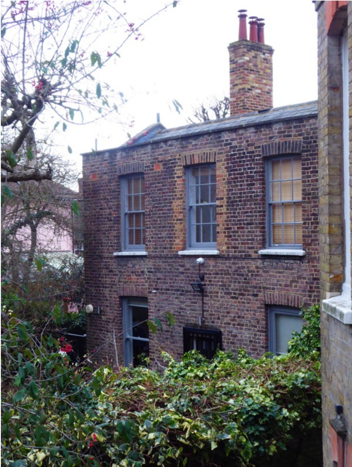
2. Rear elevation of Cossey Cottage from No 7 Pilgrims Lane
