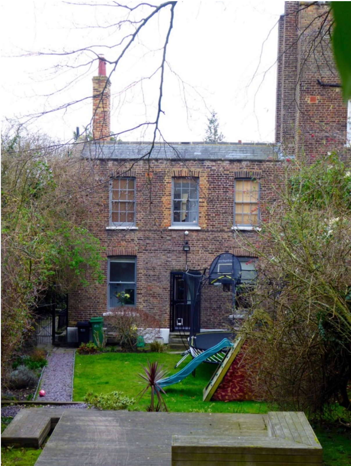
1. Rear elevation of Cossey Cottage from public grounds of Rosslyn Hill Chapel.
