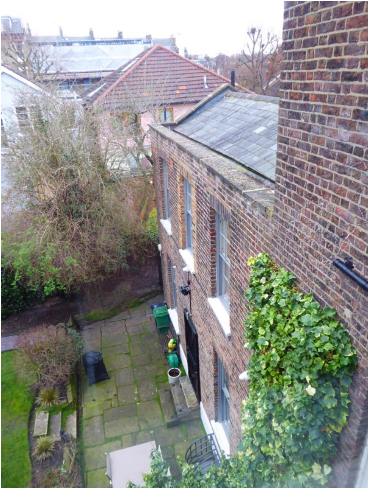
3. View of flat-fronted rear elevation of Cossey Cottage showing the position and the potential impact of a 5.5m. rear extension.
