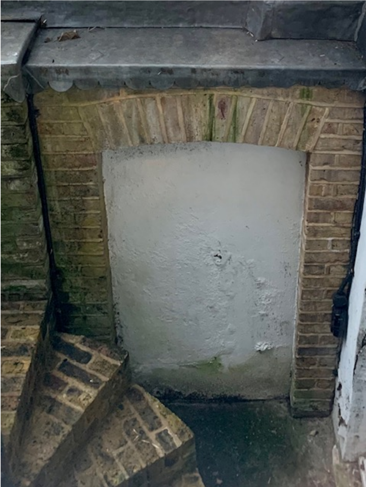
19. Bricked-up basement opening between Sidney House and Cossey Cottage
