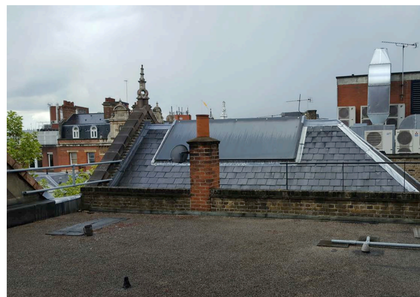
Adjacent pitched roof at 117 Shaftesbury Avenue
