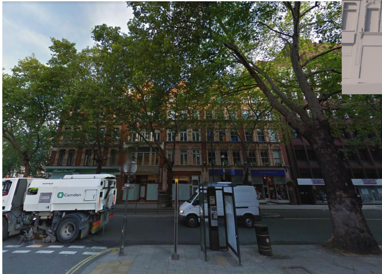
Photograph view opposite 119 Shaftesbury Avenue.
