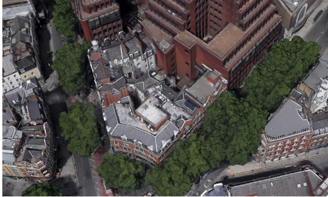
Aerial View - Facing North
