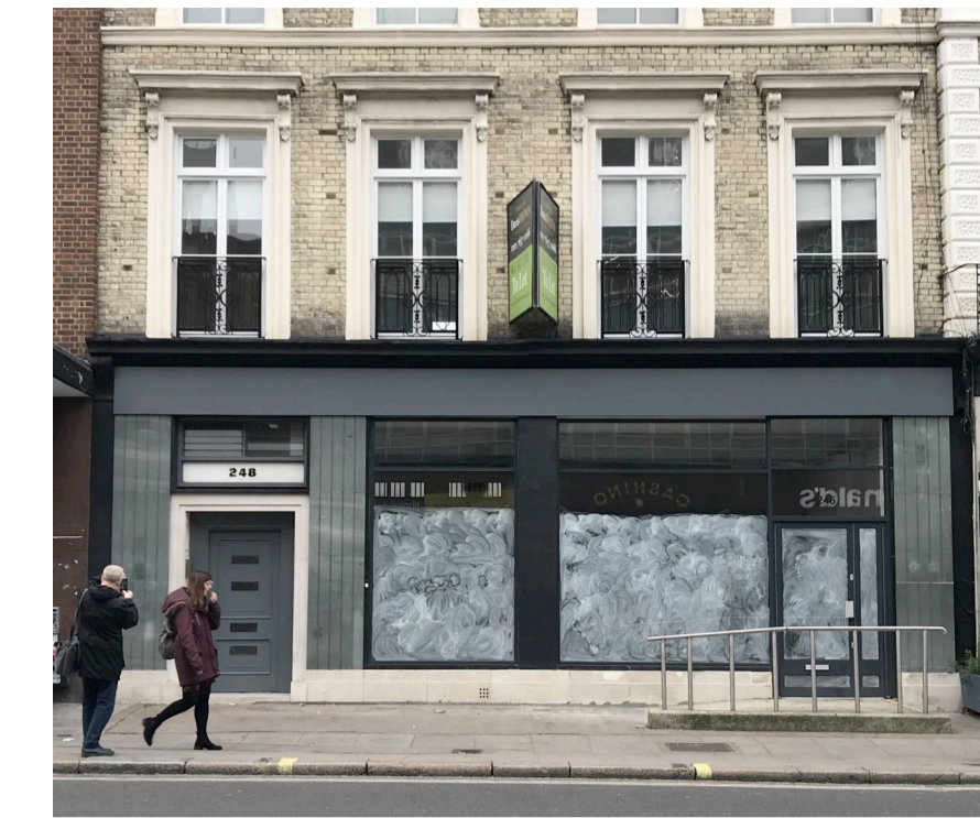
EXISTING SHOPFRONT PHOTOGRAPH
