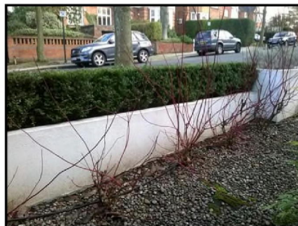
6. G4 in foreground and G5 in background
