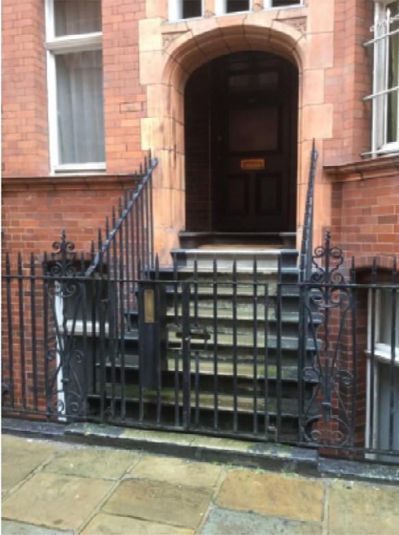
7. Non-original gates installed at foot of steps to Flat 60.
