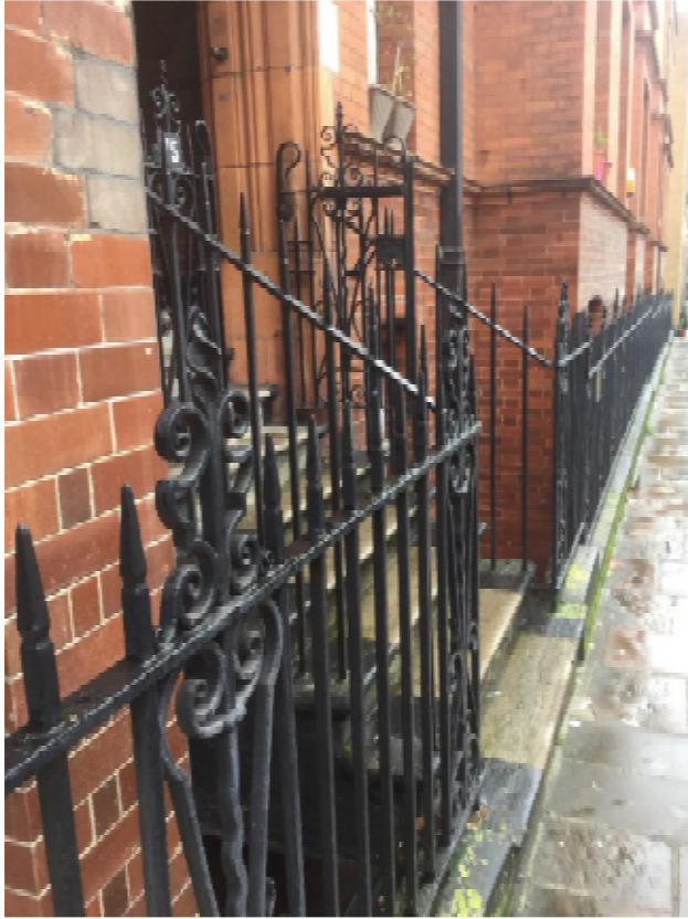
5. View of railings and steps.
