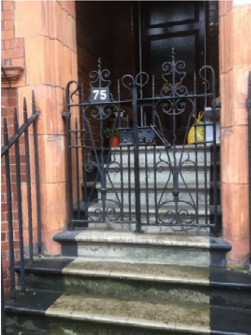
1. Existing gates in place at Flat 75 Gordon Mansions.
