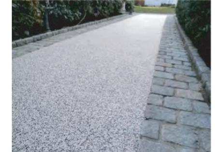
Resin-bound permeable paving
