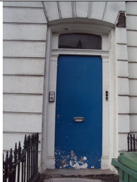
Figure 4 View of Front Door
