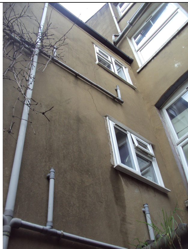
Figure 5 Rear of Property
