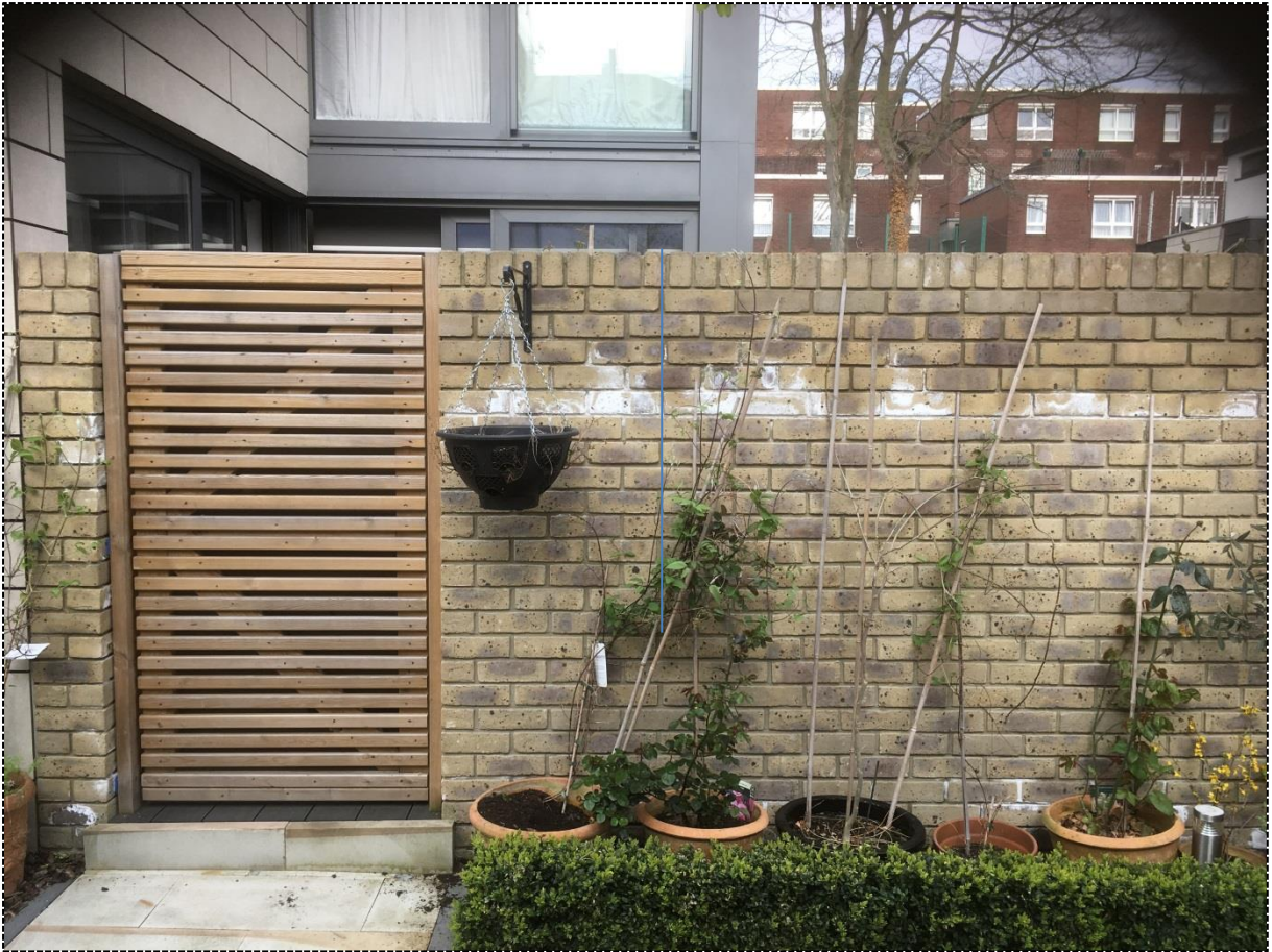
Photo.4 Side view of No.8 from footpath. Pedestrian gate to be relocated to RHS
