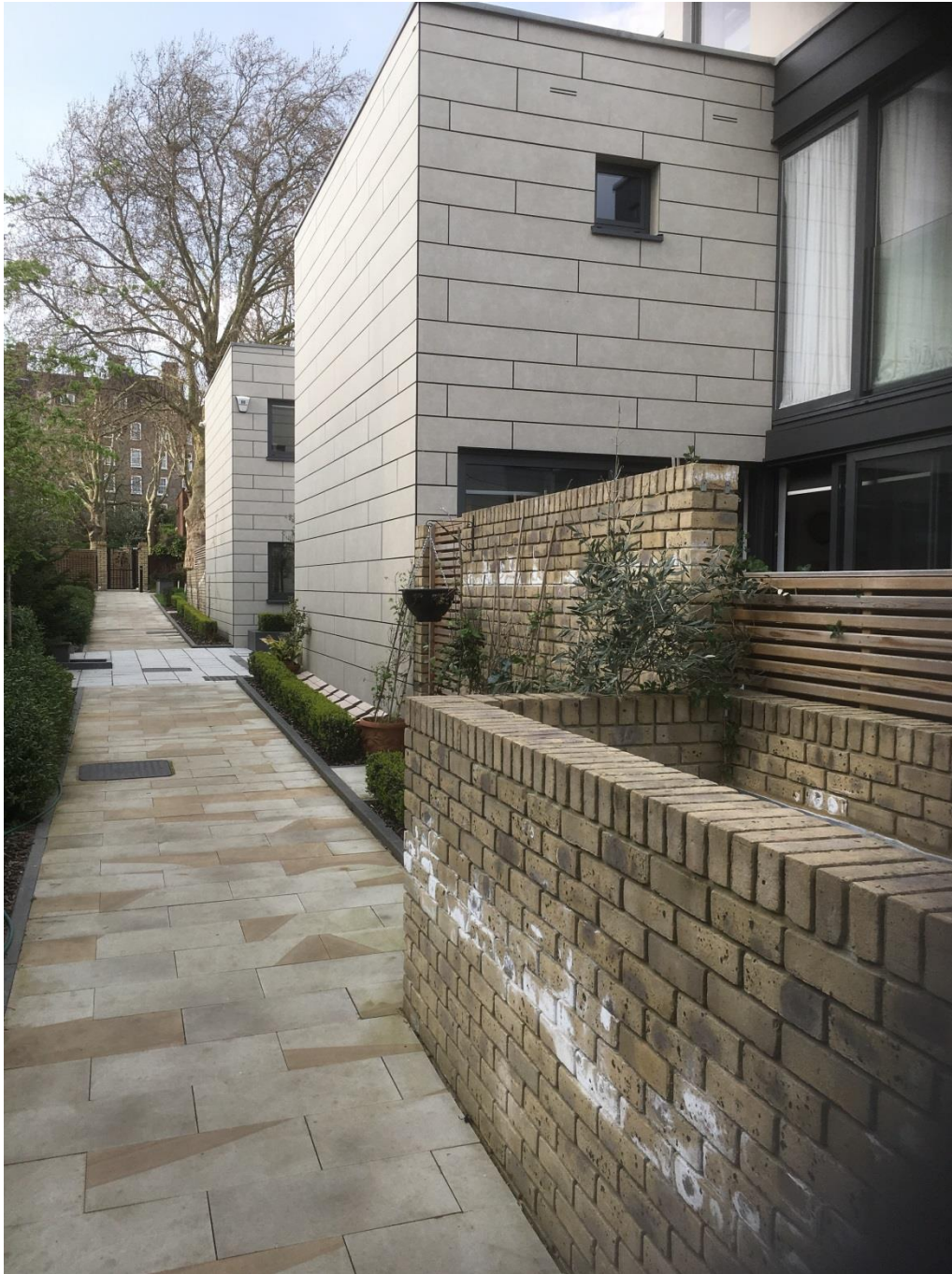
Photo.3 View from access footpath alongside College Lane.
