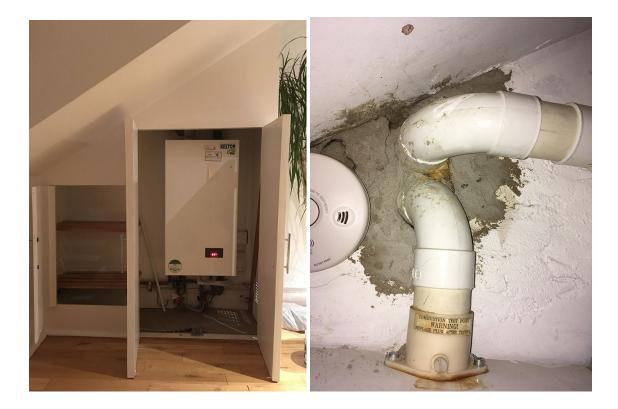
In 2008 the gas safety regulations changed requiring that the whole length of the flue is able to be examined, making use of inspection hatches as necessary (BS 5440-1:2008).
