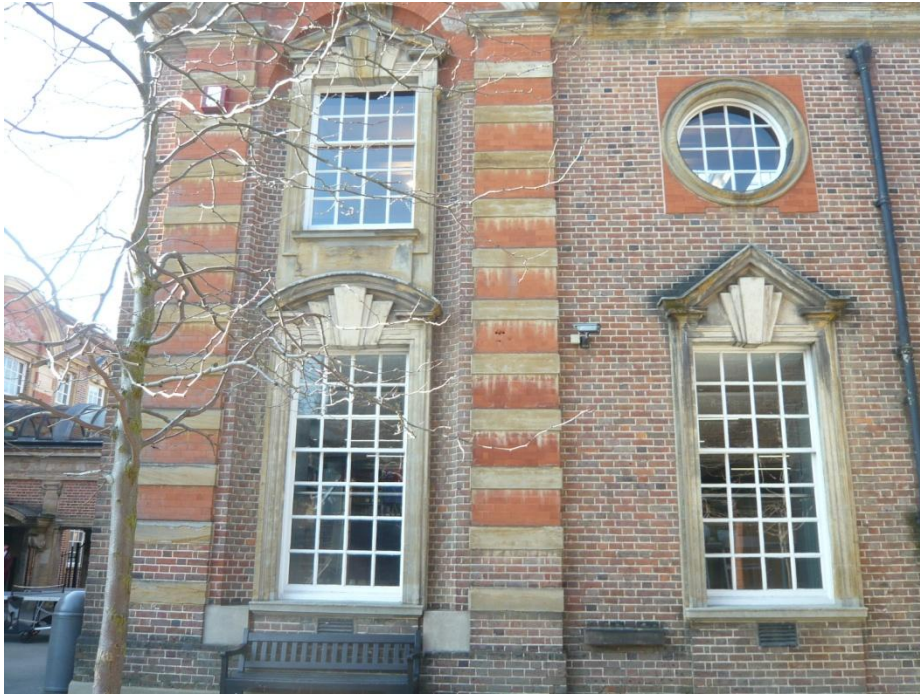
Fig.5 Close-up view of southern end of east facade of North Block
