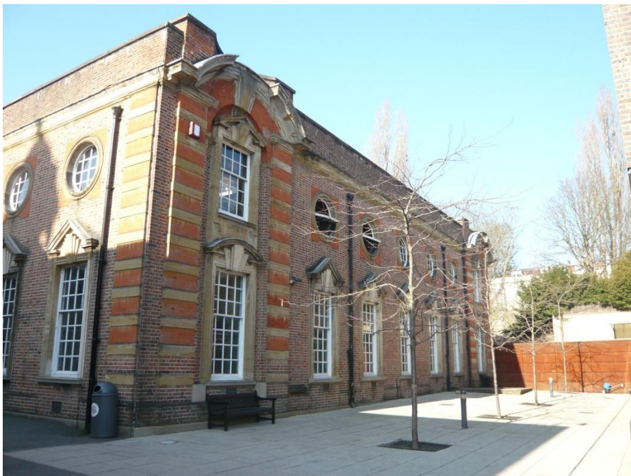
Fig.4 East facade of North Block and adjacent courtyard
