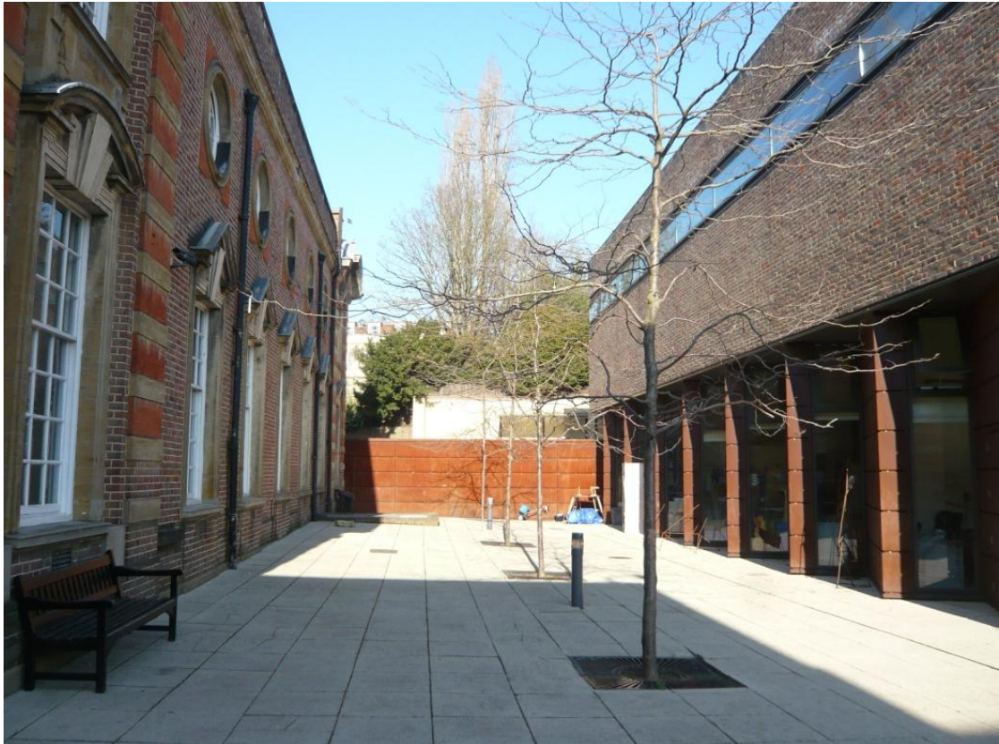
Fig.7 Paved courtyard between North Block and Bentham Building
