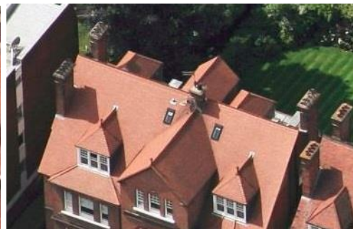
Pic. 9 - no. 15 approved rooflights
