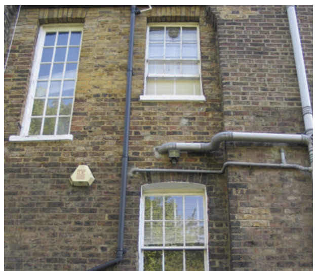
Existing SVP and waste pipes
