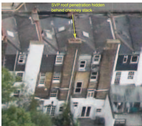
View of roof, showing proposed location of SVP
