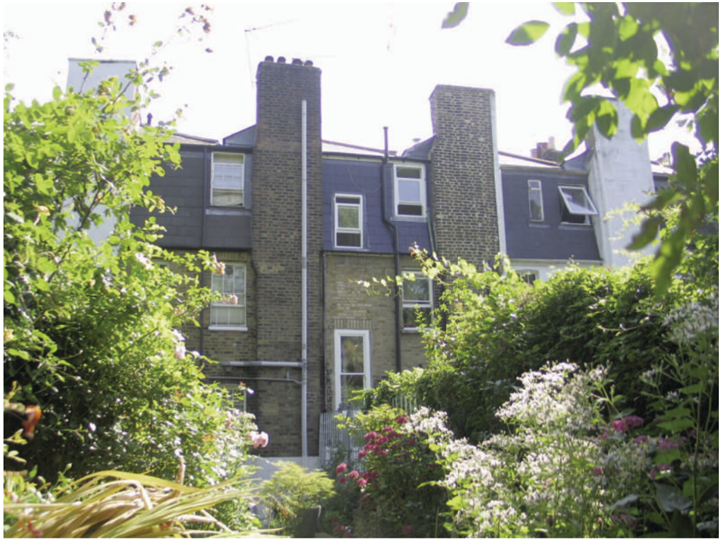
Above: view from garden of 125 No. 125 on left. Unsightly soil pipe (grey) to be relocated internally
