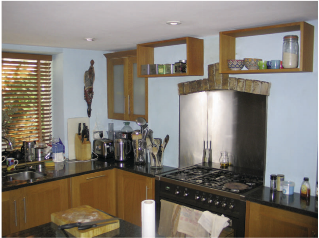
Above: Basement kitchen looking towards front Fitted kitchen to be removed and plastered wall finishes made good. Extract hood in chimney breast opening to be removed and false arch to opening to be removed.
