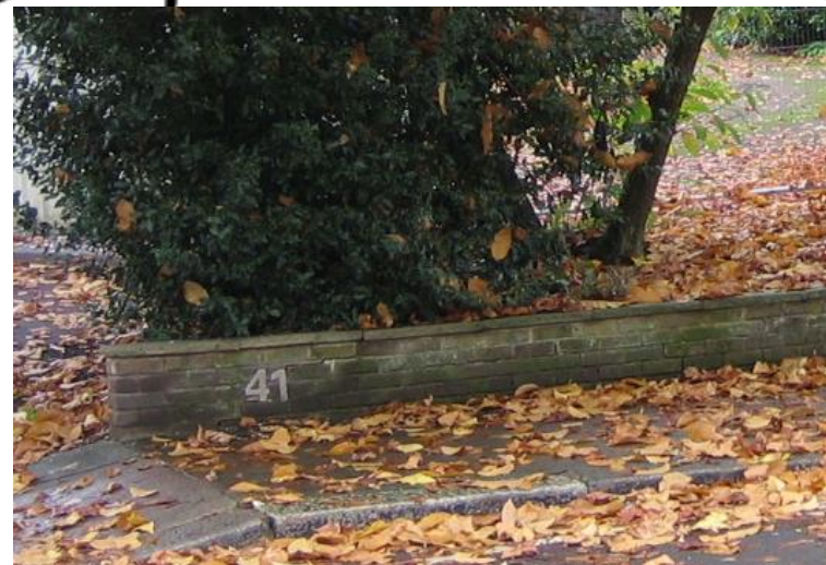
Existing low brick retaining wall.
