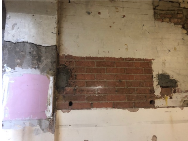
11. Detail of non-original brickwork to infill wall
