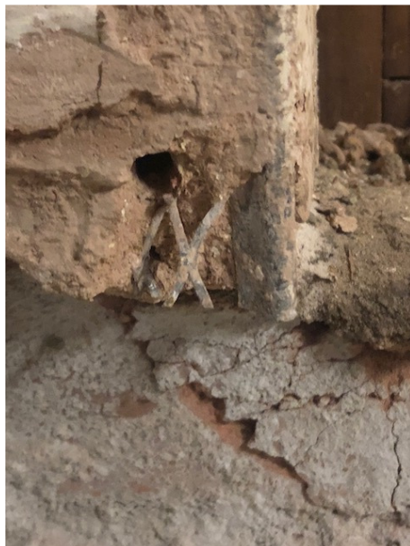
14. Detail of modern thistle plaster and metal edge bead
