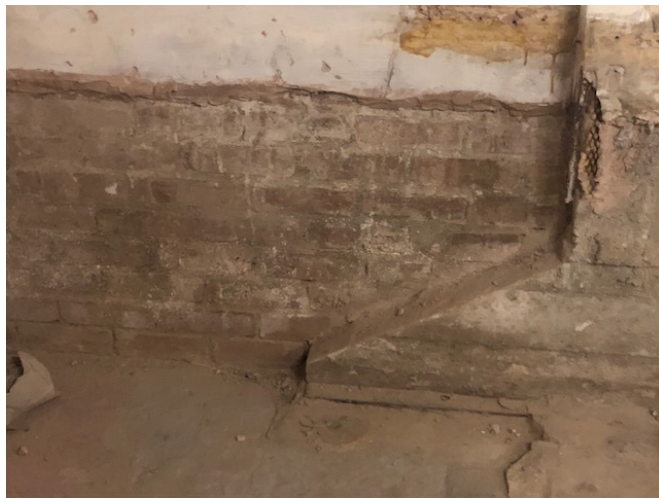
13. Detail of brickwork infill not toothed-in
