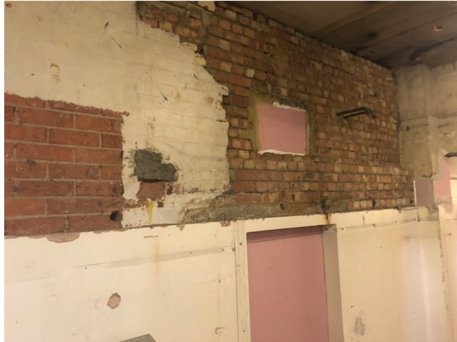
9. Detail of various brick/blockwork types to infill wall
