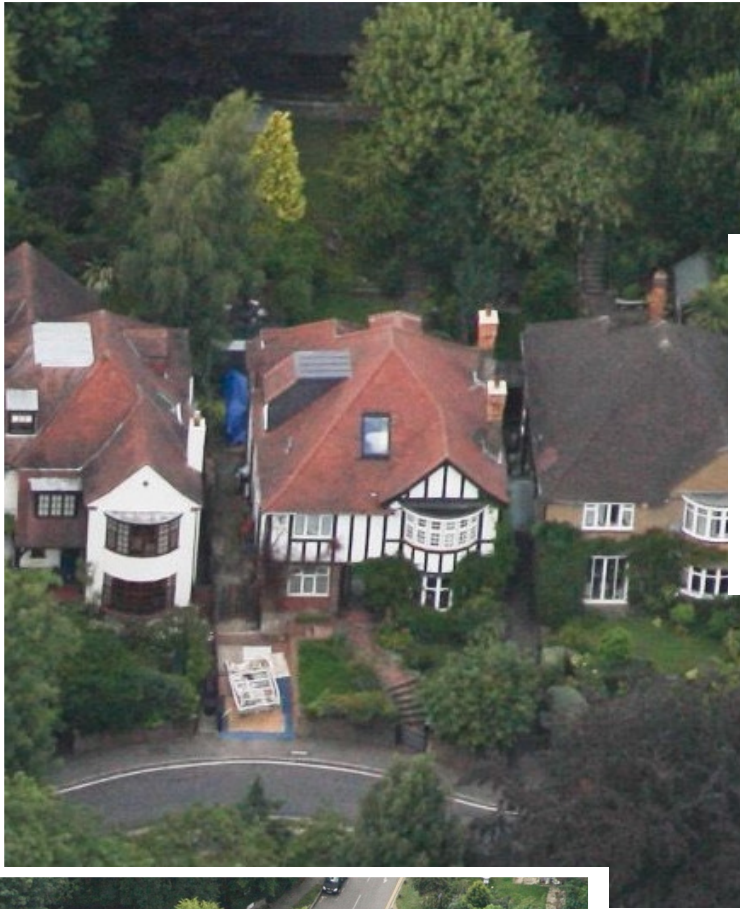
Front elevation overview image showing contextual setting of No.2 Holly Lodge Gardens
