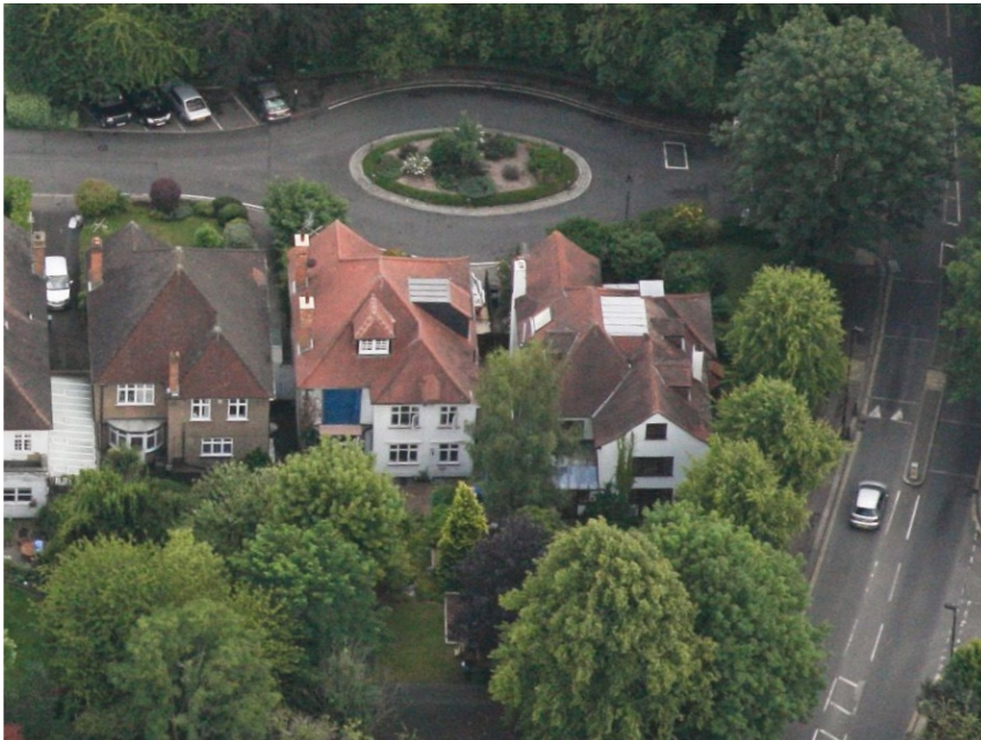
Rear Elevation overview, showing rear ground floor extension to No.1 Holly Lodge and deeper rear building line.
