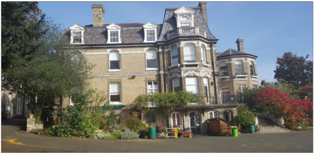
2. Existing view of south elevation
