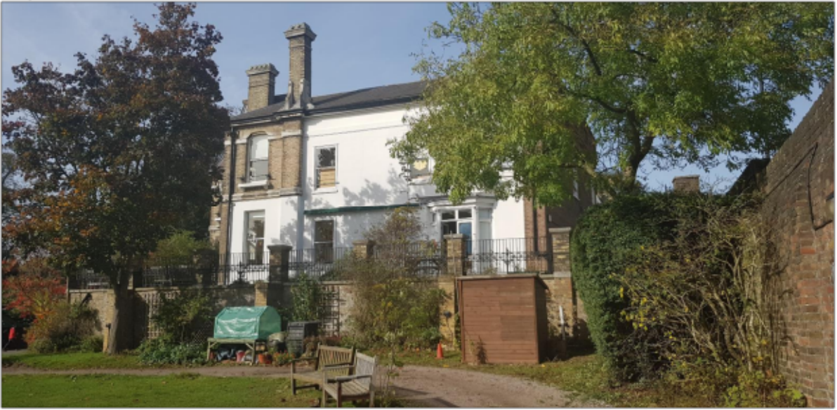
3. Existing view of east elevation
