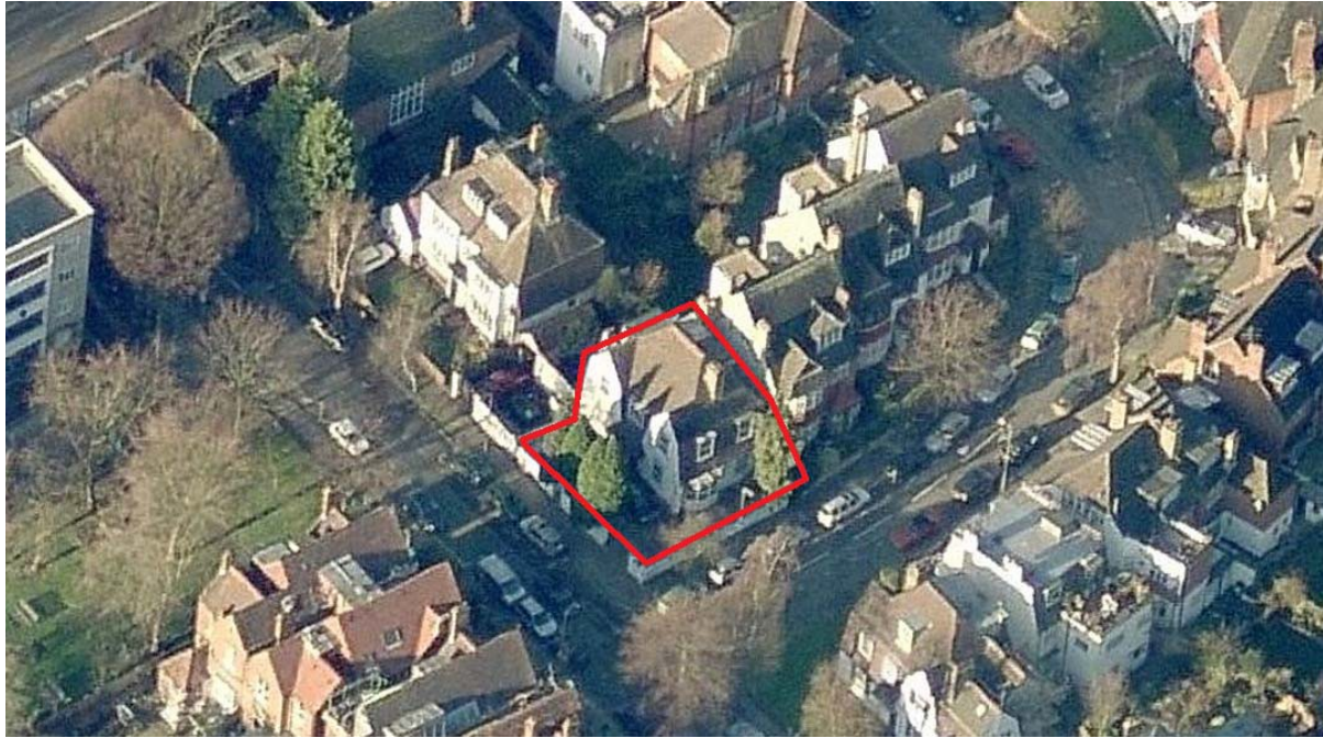
Arial View of Site Image Courtesy of Bing Maps
