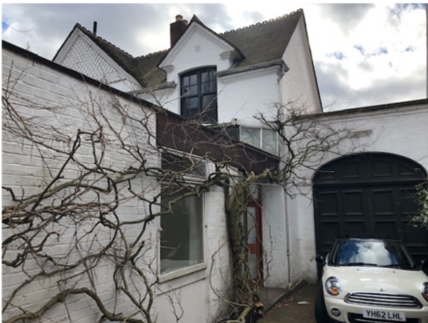
3) Front/side elevation from within the driveway
