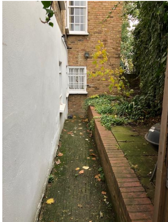
3) Existing side access
