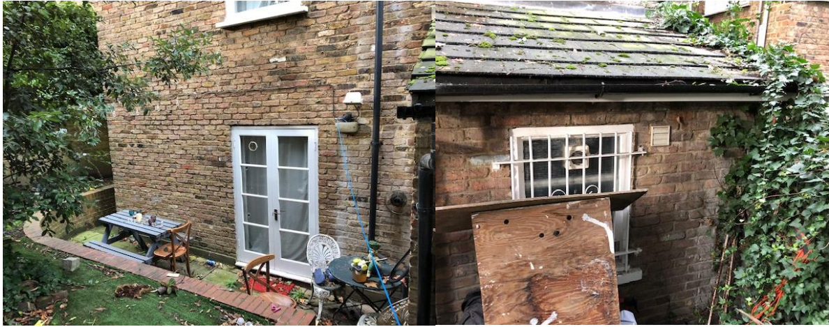
1) Rear elevation of the property with existing excavated patio and single storey outrigger
