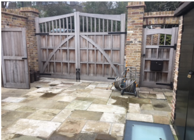
View of gates internally
