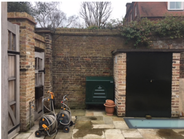
View of gate/store area
