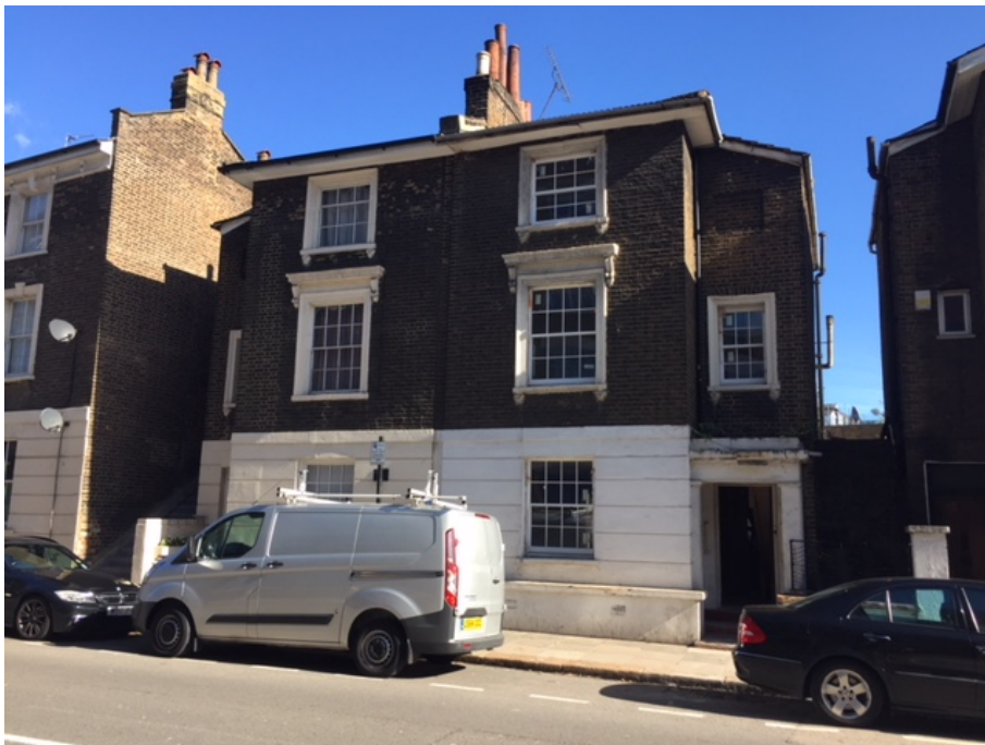
Photo 2 (above): Front elevation of Nos. 70 and 68 Highgate Road
