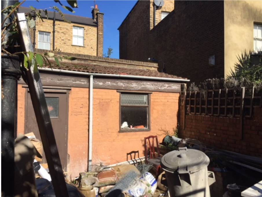
Photo 7 (above): Existing single storey rear closet wing (looking north)
