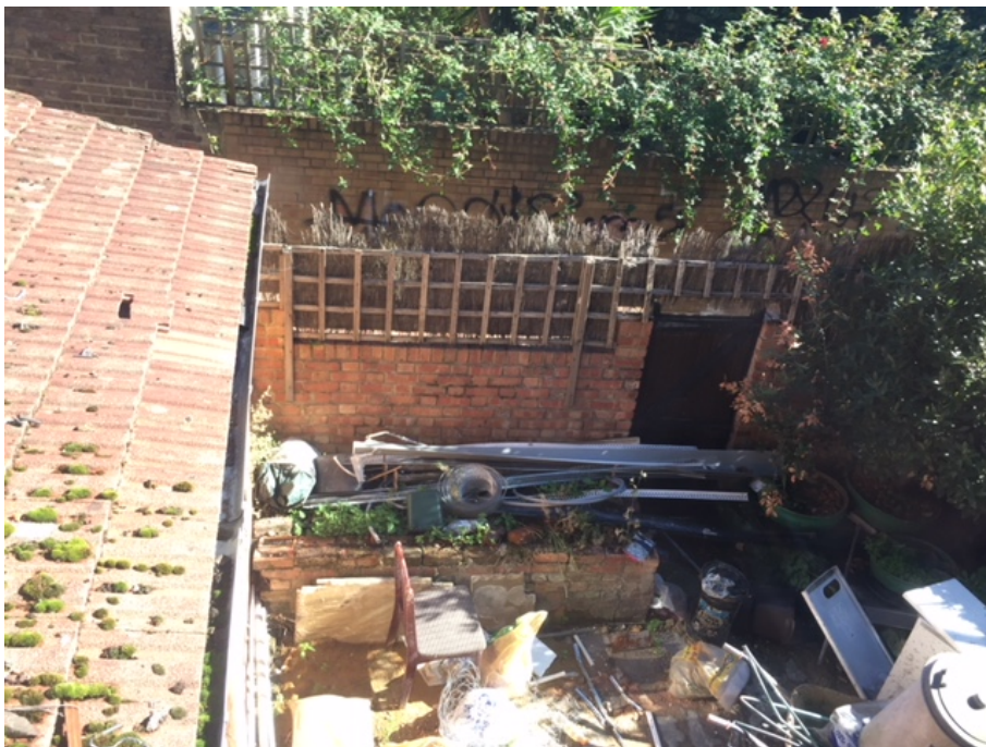
Photo 10 (above): View of existing rear courtyard and rear boundary wall
