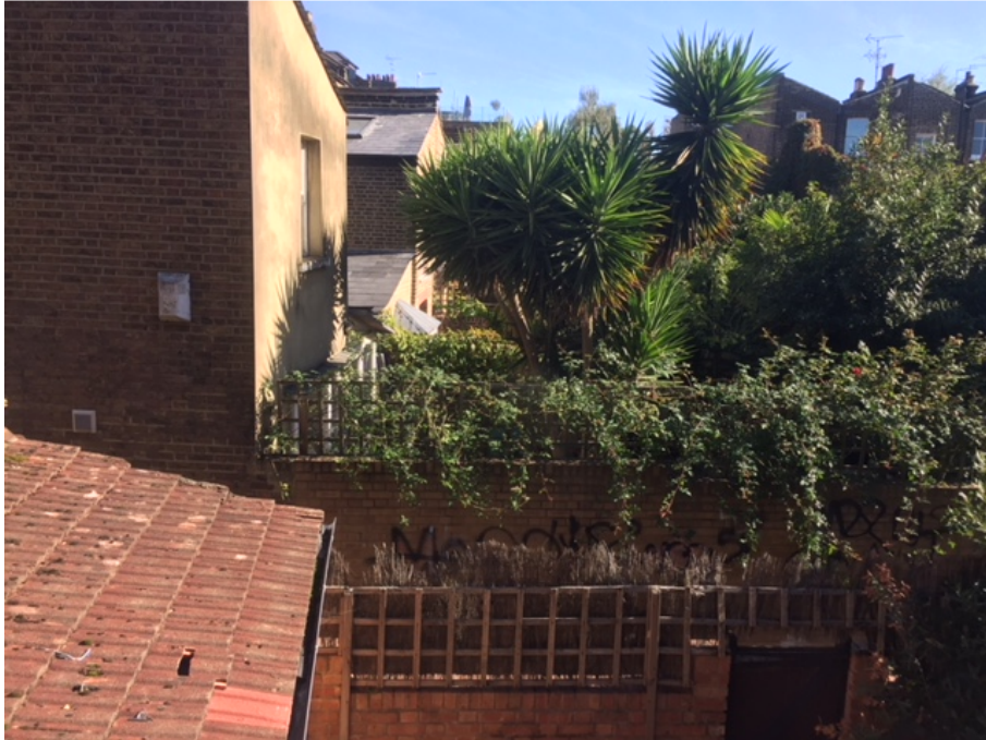
Photo 11 (above): View of rear boundary wall and College Lane to rear of property
