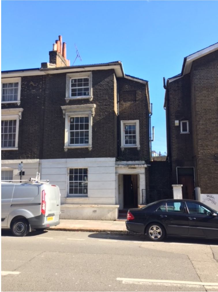
Photo 1 (above): Front elevation of No. 68 Highgate Road
