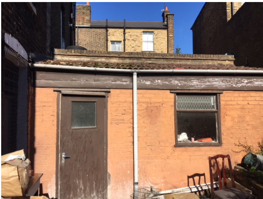
Photo 8 (above): Side (south-eastern) elevation of existing rear closet wing
