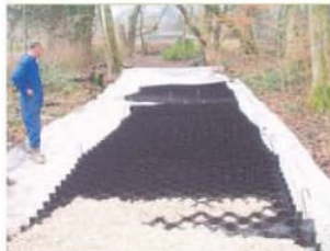
CellWeb during installation.
