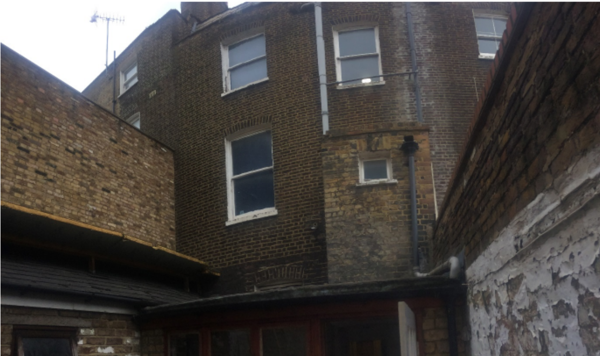
4. Existing rear elevation of no. 110
