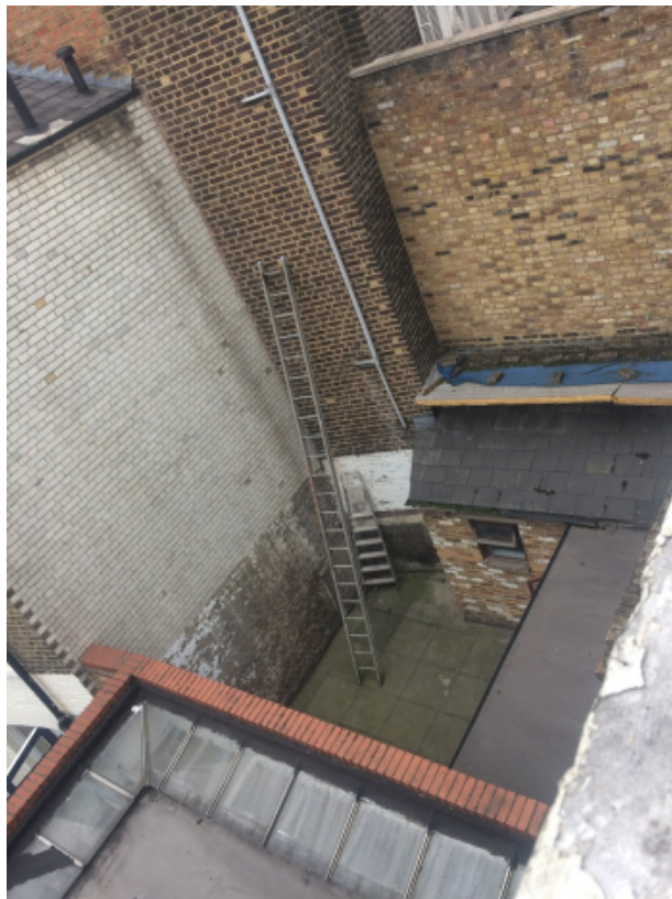
6. View of rear courtyard at no. 110 from roof level; single storey rear structure to be partially demolished.
