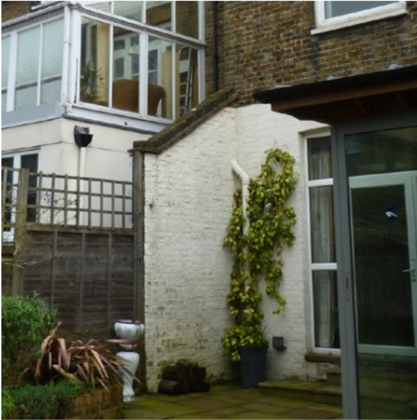
3. Existing boundary wall with no. 58 Dartmouth Park Road.
